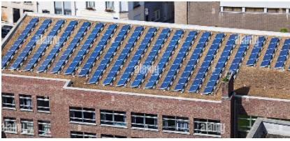
Solar Panels Roof Example
