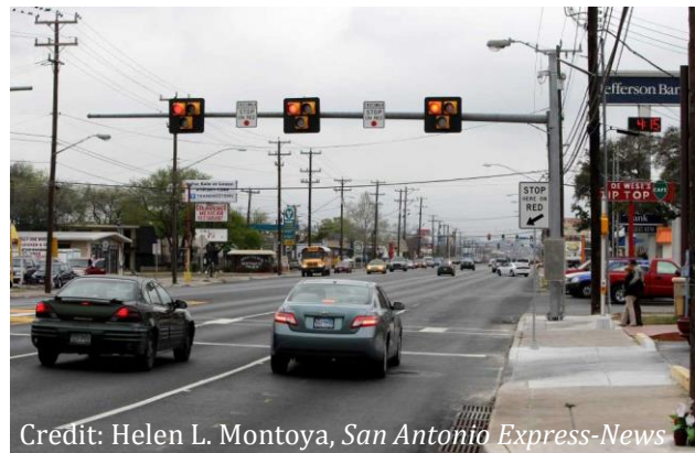
Figure 12. This High Intensity Activated Crosswalk (HAWK) is located on Fredericksburg Road north of Santa Anna Street in San Antonio, TX
