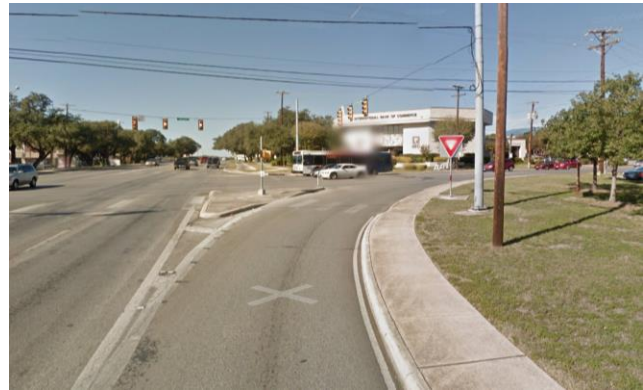
Figure 9. Large turning radii increase pedestrian crossing distance and enable vehicles to turn at high speeds
