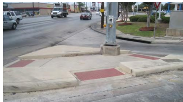
Figure 10: A right-turn slip lane with directional island (top) should provide adequate space for people using wheelchairs and strollers as in this example
